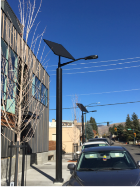
Above and Below: Inovus Element Plus solar-powered shielded street light in public right of way, Ketchum.
