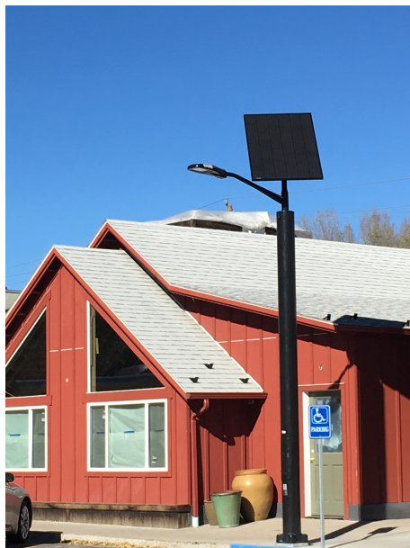
Above and Below: Inovus Element Plus solar-powered shielded street light in public right of way, Ketchum.
